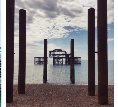
Array Structural Support
